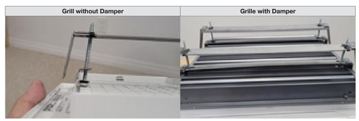
**NOTE:** If the grille has a mounted damper, fully open the damper blade.
